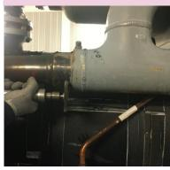
Apply a half shell on the piping to make sure here is no roughness left
