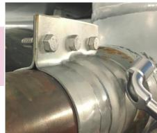
Now you can clean the excess of glue and start the circuit, the glue takes 30 minutes to harden with 60°C discharge temperature (or 8h with stopped unit at 23°C)
