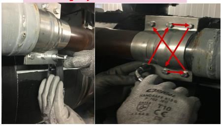
Screw until the nuts are hardly tightened as well as the edges of the shell
